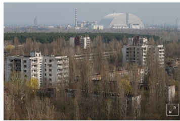
A New Safe Confinement (NSC) structure over the old sarcophagus covering the damaged fourth reactor at the Chernobyl nuclear power plant is seen from Ukraine's abandoned town of Pripyat, Ukraine, April 5, 2017. REUTERS/Gleb Garanich
